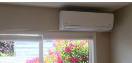
Mini-split air-source heat pump – indoor head
