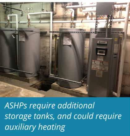
ASHPs require additional storage tanks, and could require auxiliary heating
