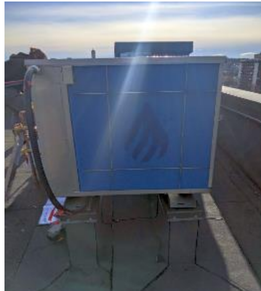
Example of R410A heat pump hot water system mounted on the roof.
