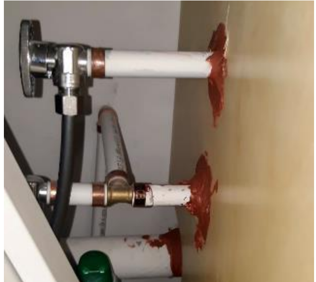
Typical firestop caulking retrofitted to seal air leakage
