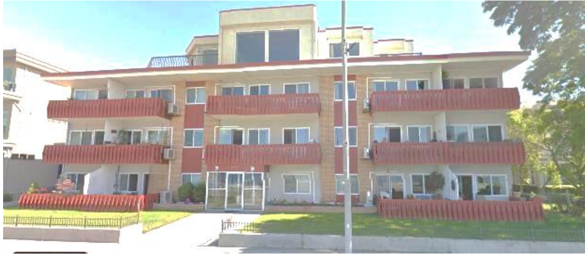
Example of mini-split heat pumps on balconies; used for summer air conditioning, spring and fall heating to complement high temperature hydronic system for peak winter heat. (Image credit: Google Maps)
