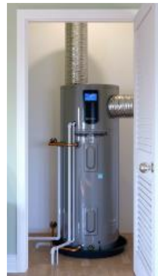
Tank type heat pump water heater (HPWH); suitable for in-suite use located in a closet.
